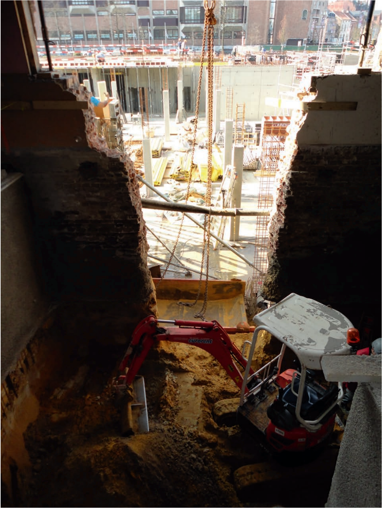
BREACH FOR CONNECTING CORRIDOR
