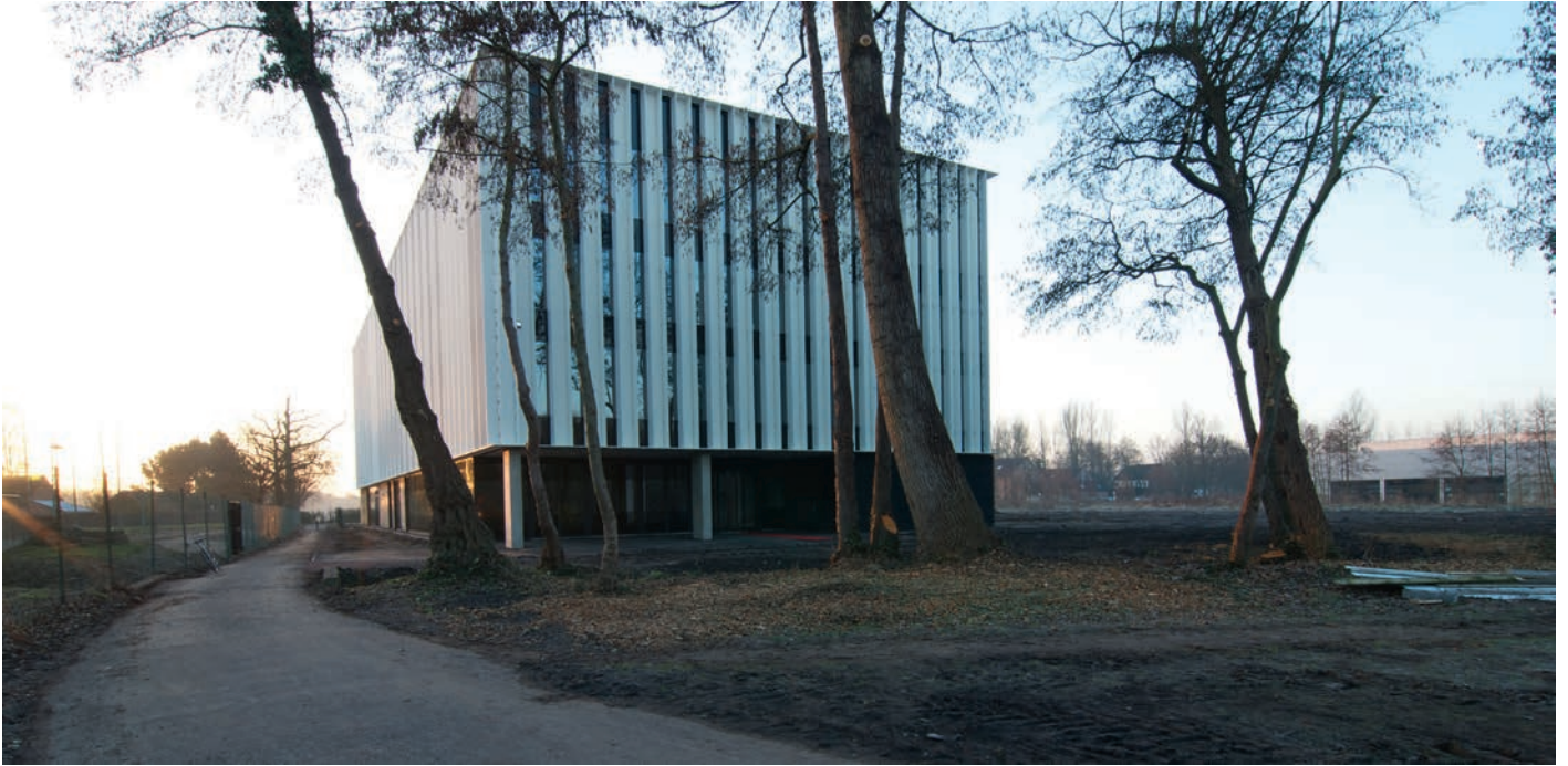
NEW KHLIM BUILDING, DIEPENBEEK
