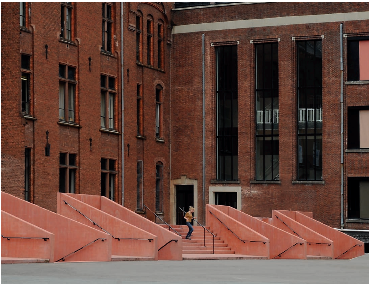
ACCESS STAIRS TO SANITARY FACILITIES. PHOTO: ELISE VANHEES
